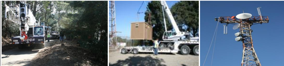
Skyline shelter delivery and antenna installation
