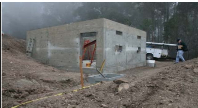
UC BERKELEY SHELTER- PROGRESS
