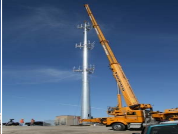
PATTERSON PASS MONOPOLE TOWER COMPLETE
