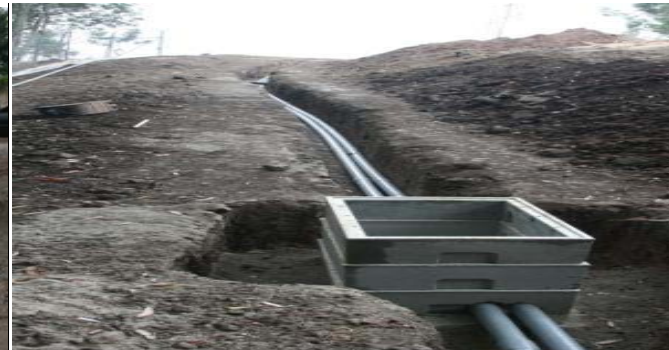
UC BERKELEY TRENCH FOR POWER AND DATA
