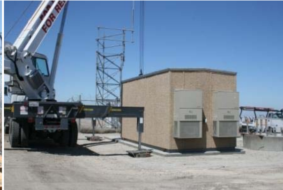
PATTERSON PASS SHELTER INSTALLATION
