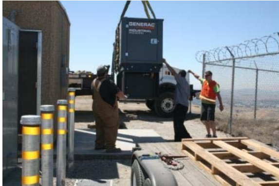
PATTERSON PASS GENERATOR INSTALLATION
