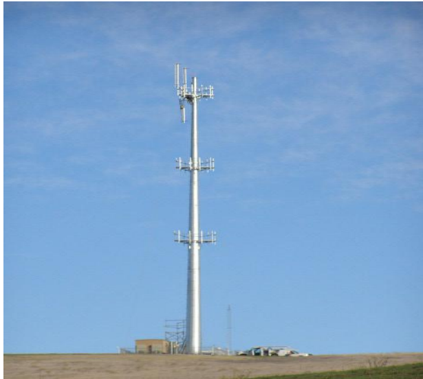
PATTERSON PASS SITE
