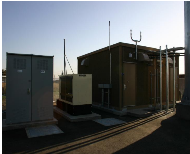
Warm Springs Completed
