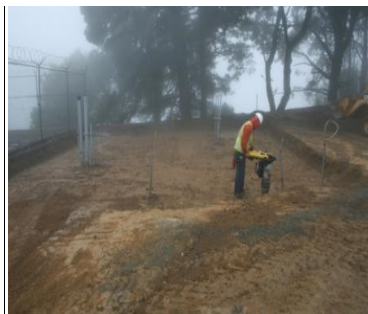
SKYLINE SITE PREPARATION
