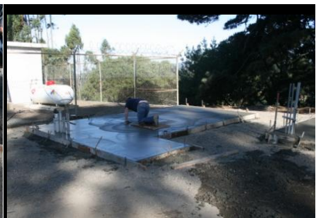
SKYLINE SHELTER FOUNDATION
