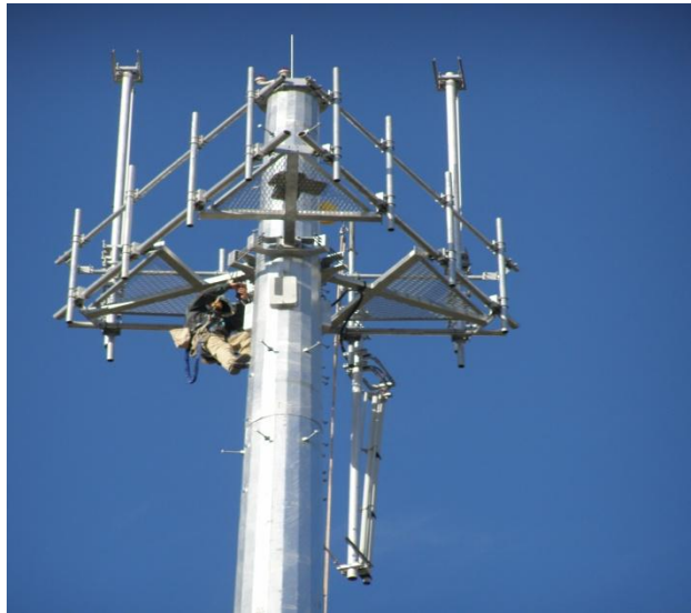
PATTERSON PASS MONOPOLE TOWER COMPLETE
