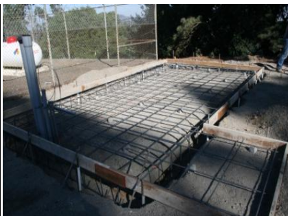
SKYLINE SHELTER FOUNDATION
